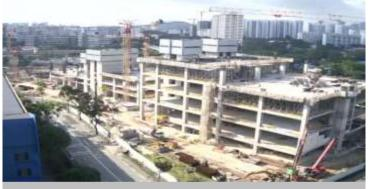
Completed level 4 casting in Block 1; level 2 casting in Block 2; and level 1 casting in Block 3
